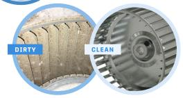
"1/8 of an inch of dirt and dust build-up on the blower wheel can reduce airflow by up to 30%"
