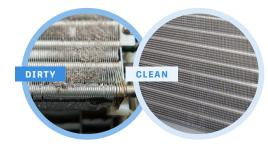
"0.25 mm [1/100 of an inch] of buildup of dust on an evaporator coil can result in a 20% decrease in system efficiency." — Prism Engineering
