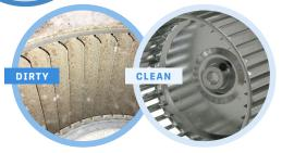
"1/8 of an inch of dirt and dust build-up on the blower wheel can reduce airflow by up to 30%"
